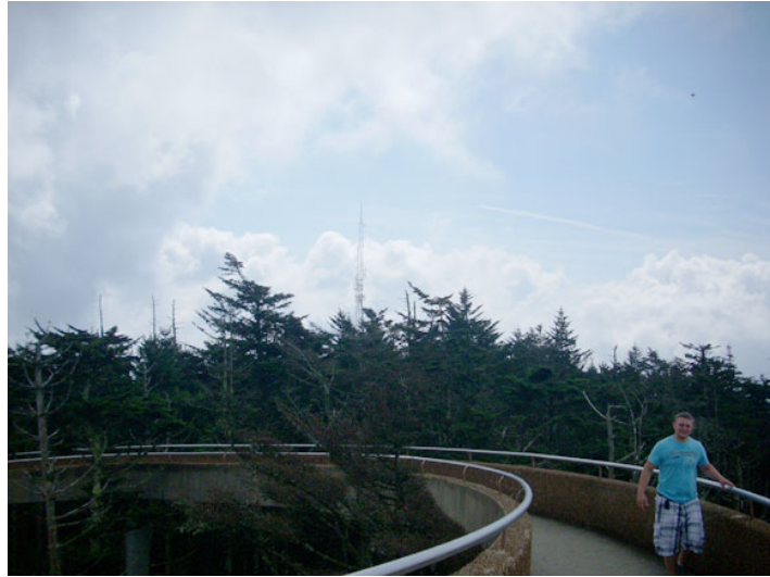
Figure 2: Elevated walkway at Clingman's Dome.
